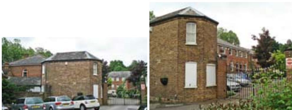
The former entrance lodge is situated by the gates of King George Square.
